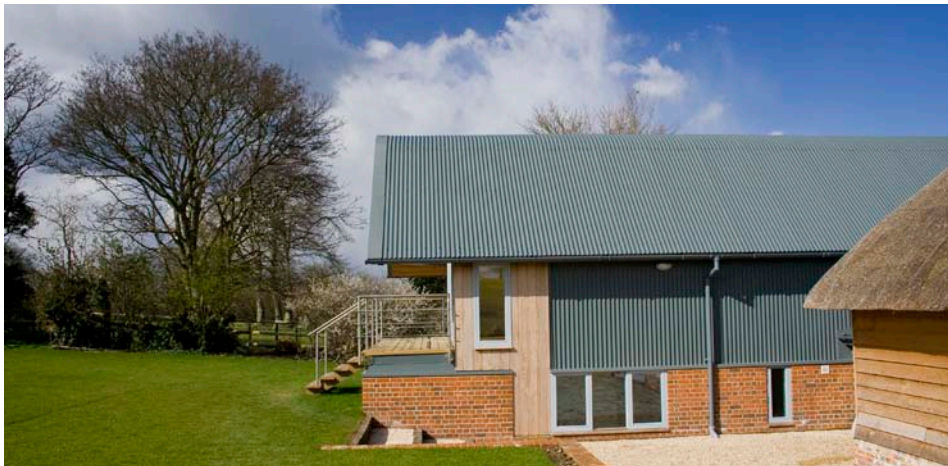
Above Externally, natural materials of the original barn contrast with the crisp appearance of the new wing Left The projecting canopy becomes even more dramatic after dark Below The newly repaired barn dominates the overall composition.
