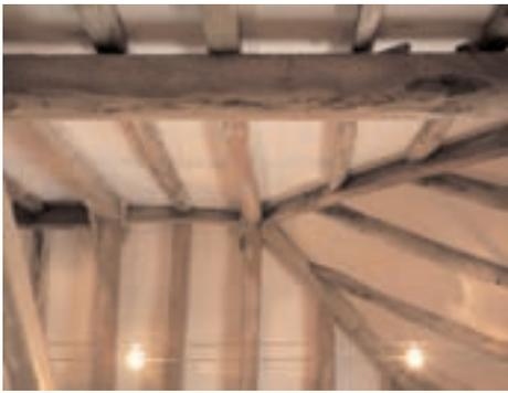
At first floor, lighting is provided in the form of a tensioned wire system running beneath the ridge of the roof structure. Again this arrangement allows an infinite degree of flexibility in lighting placement, while remaining independent of the roof structure itself.
